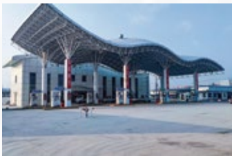
The Puyang Integrated Energy Station, which includes oil, hydrogen, gas, and electricity, is the first in Henan Province to have both 35MPa and 70MPa hydrogen refueling capabilities.
