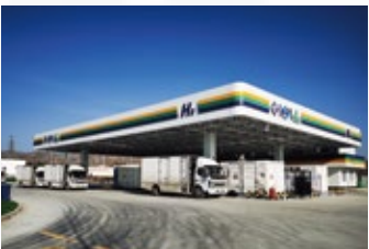
The Chuangba Hydrogen Refueling Station, built in 2018, served the 2022 Winter Olympics.
