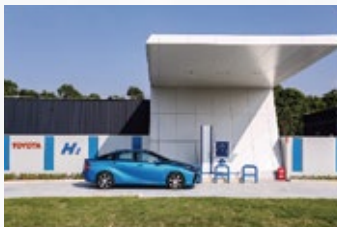
Toyota's first hydrogen refueling station in China, and the only one in the country fully compliant with the SAE J2601 standard for 70MPa hydrogen refueling.
